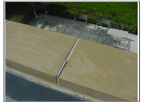
No DPC to coping stone a way around this would be capping the coping stone or removing it and adding a DPC and replacing it with a suitable coping stone.
