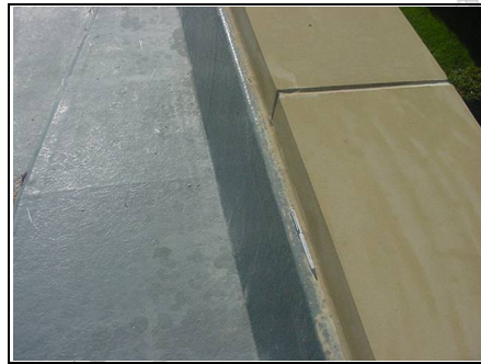
No drip detail to the front of the coping stone allowing water ingress into the property
