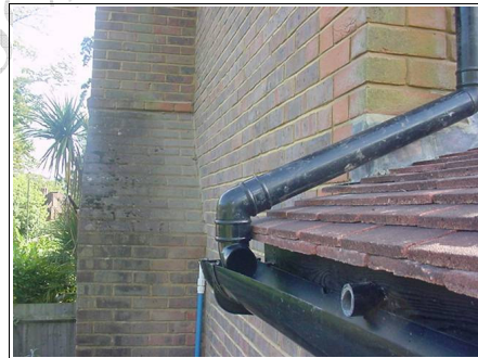
Overflowing to the rear right hand side
