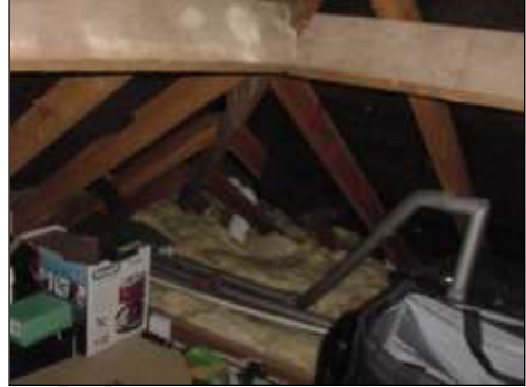
Insulation to roof with part of the roof boarded over
