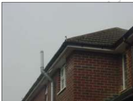
Vented soffit to the side
