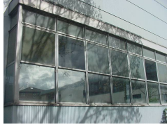
Older style windows
