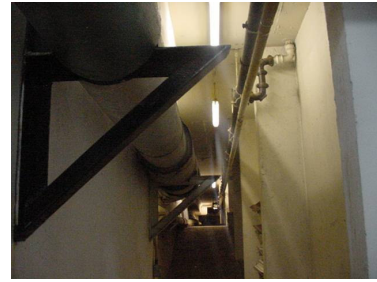
Rear of plant room
