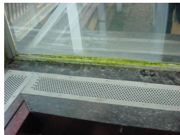
Curtain wall between gym and swim pool with moss visible at ground level
