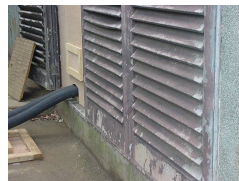
Plant room doors
