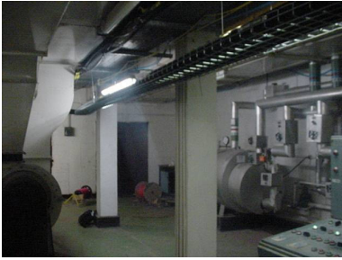
Front of plant room
