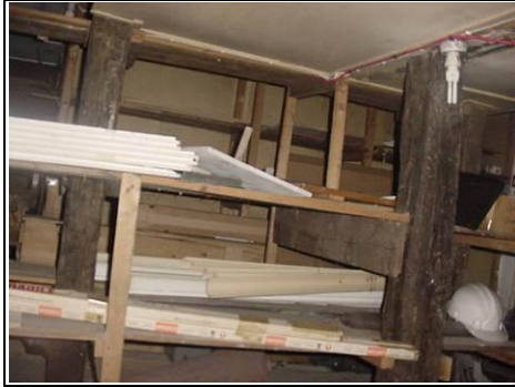
Back of basement
