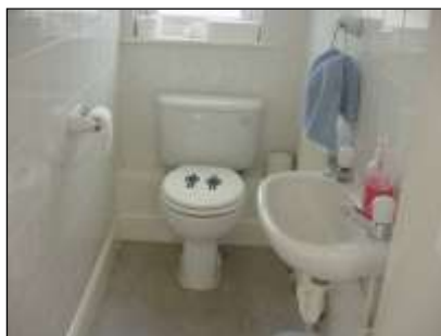
Clients' Toilets One
