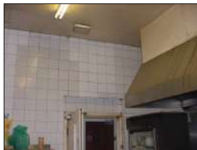
Tiled wall in Kitchen
