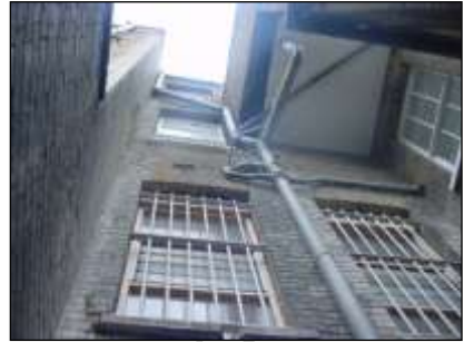
Close up of rear
