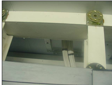
Low level firebreak
