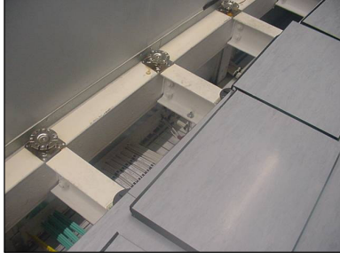
Floor panels lifted
