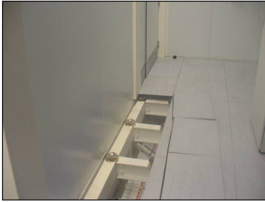
Three floor panels lifted
