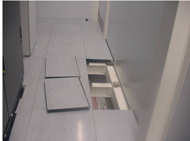
Two floor panels lifted
