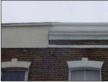
A close up of the front parapet wall, left hand side
