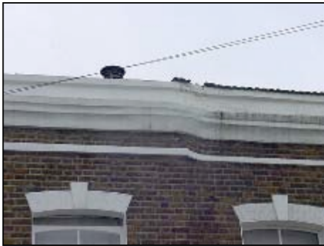
A close up of the front parapet wall, right hand side
