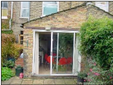
Base of the Property
