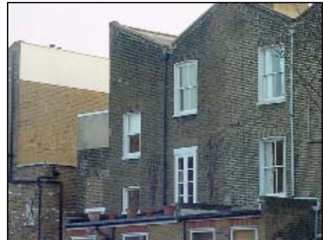
A closer view of the rear elevation
