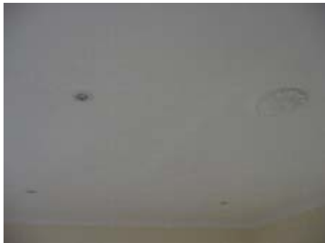
Ceiling lights to your property
