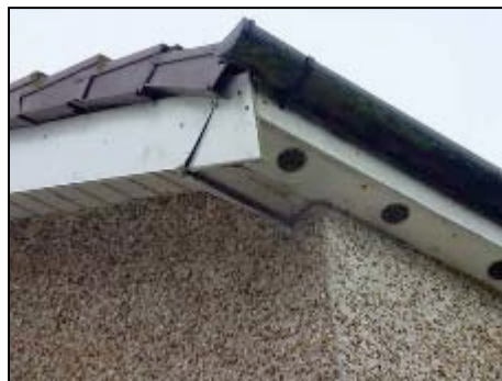
A view of the fascia and soffits boards.
