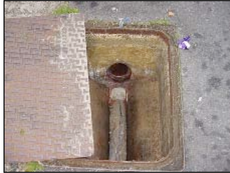
Inspection chamber at the end of the drive.
