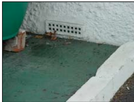
An airbrick to the front of the property
