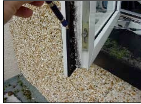
This for example is to the rear right hand bedroom window.
